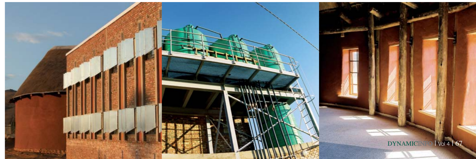
Round adobe multi-purpose classroom & solar shading on west facing windows
